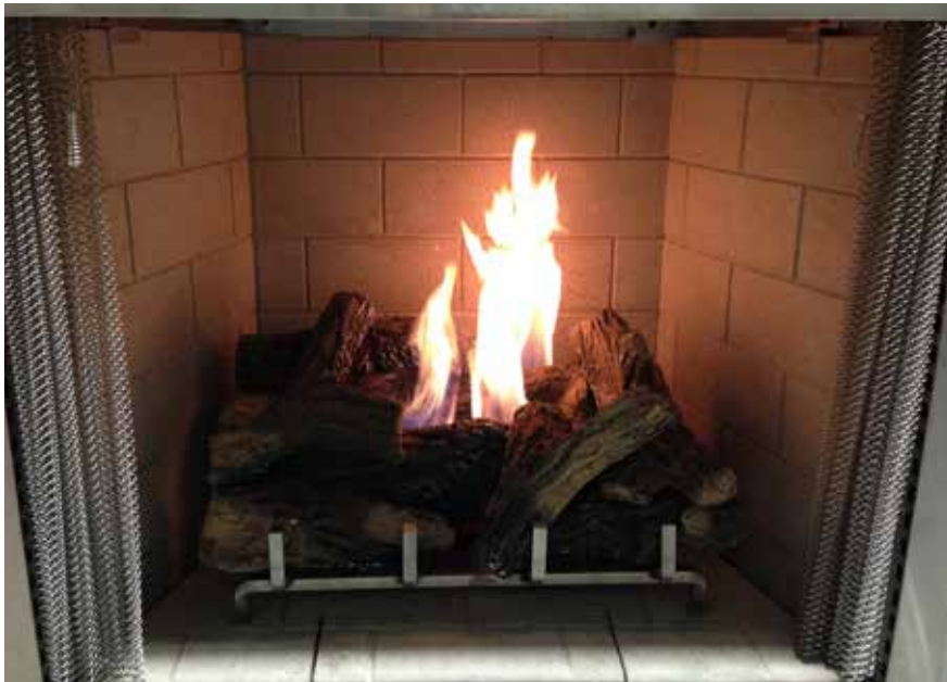
Figure 23 - Proper Burner Flame Appearance
